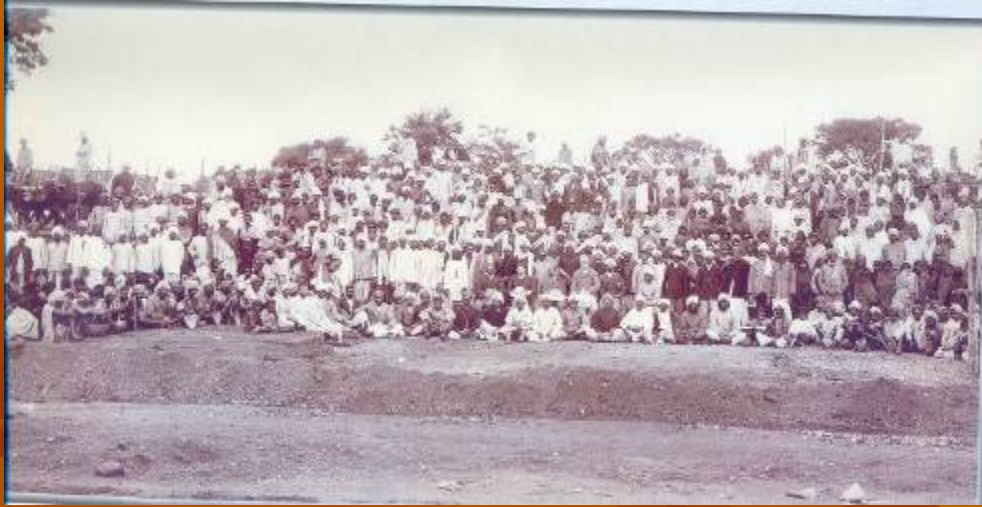
Picture of Construction Workers
