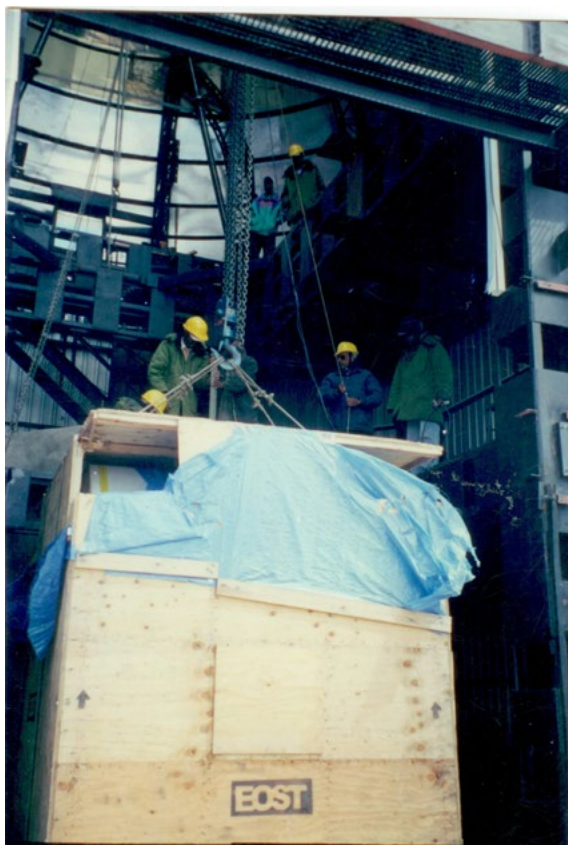
Mirror box being lifted to top floor inside the dome
