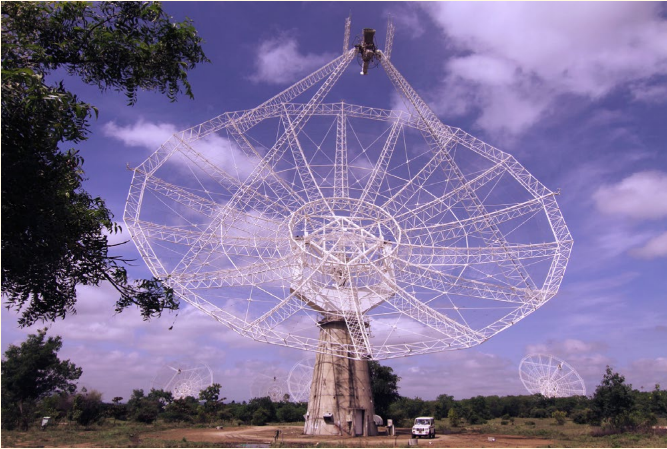
Close-up view of a 45m parabolic dish antenna of the GMRT. (Image Credit: NCRA archives)
