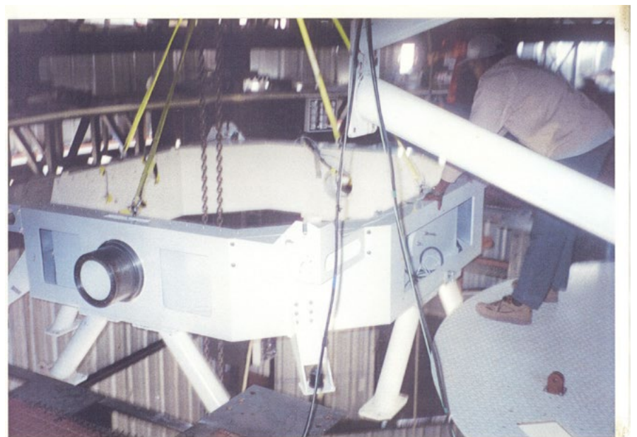
Mirror support system being fixed above pier
