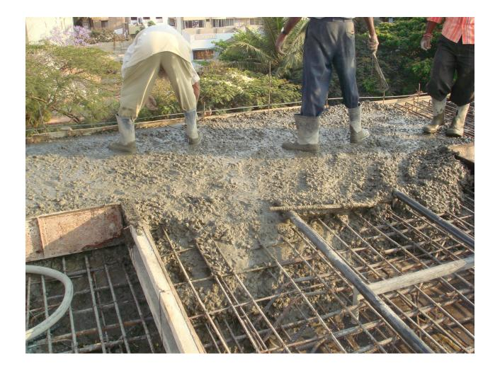
Over vibration and under vibration is harmful and should be avoided. Over vibration causes separation of coarse aggregates towards the bottom of the form and cement slurry towards the top. Inadequate compaction leads to honey- combing
